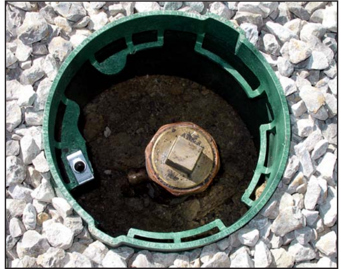
Chem-Rod grounding electrode installed in service well.
